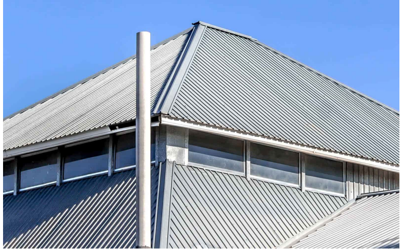
Finished galvanized metal roofing
