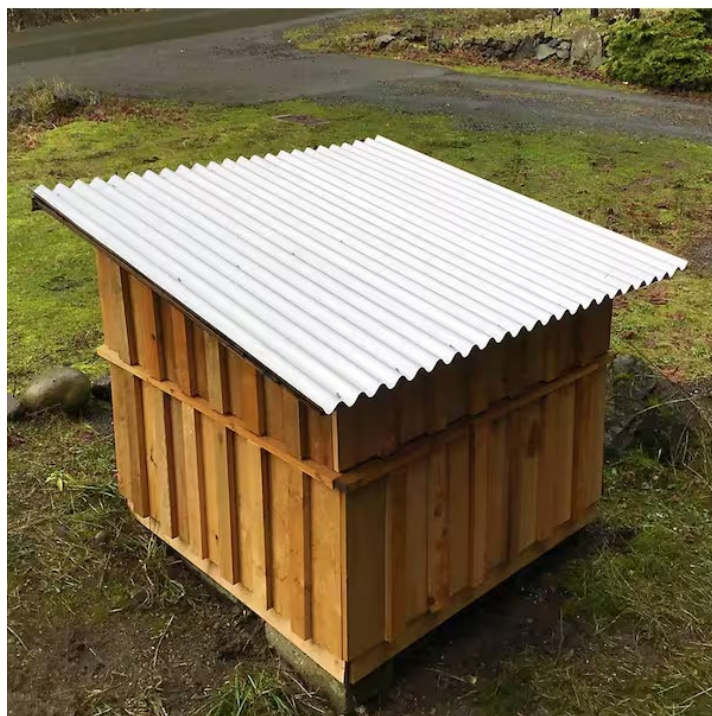
Corrugated/Unfinished metal roofing
