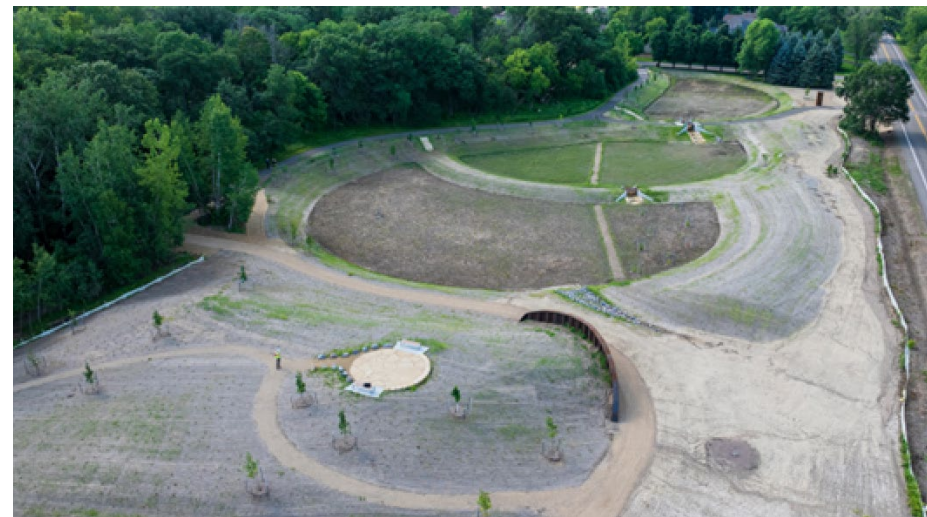
Hassenbank Stormwater Park – Woodbury, MN
