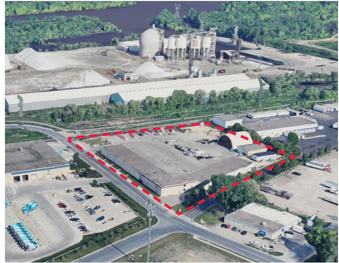
Existing facility and site, view from NW.
