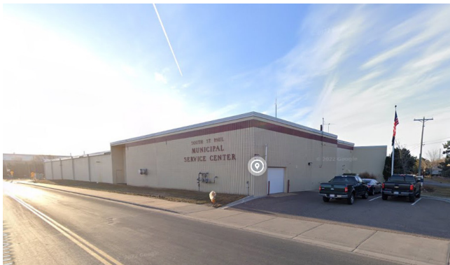
Existing facility from Richmond St
