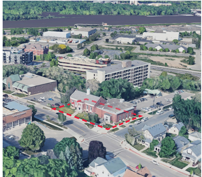
Existing facility and site, view from SW.
