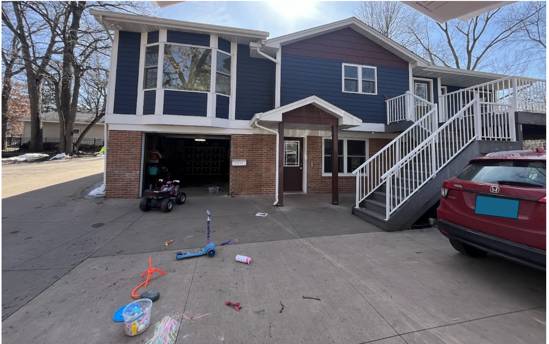
Photo of the Front Façade and Single Stall Garage of 1820 Faber Avenue
