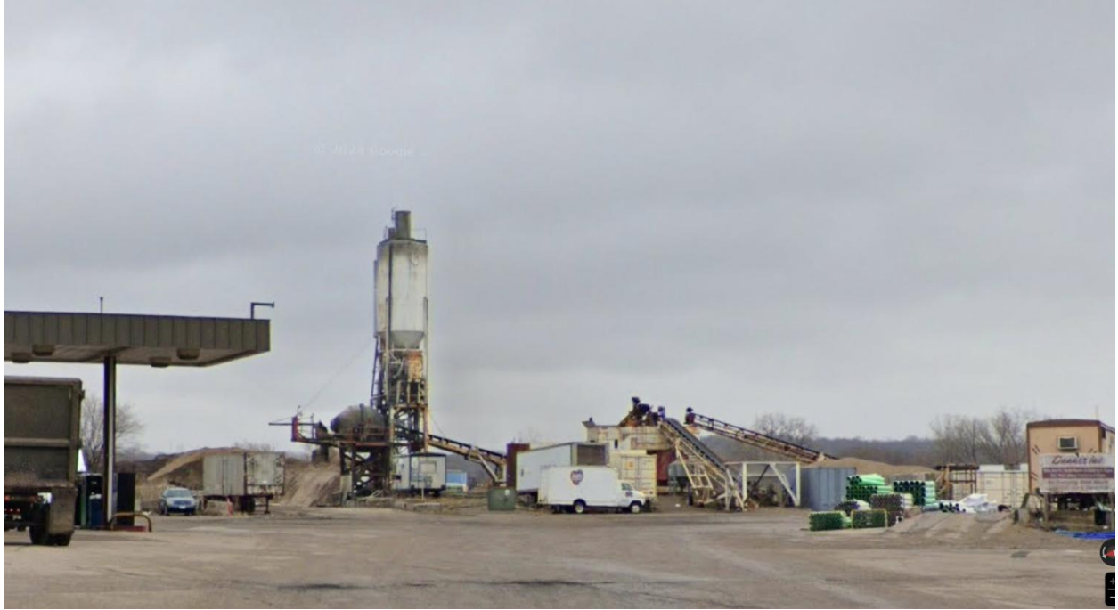
EXISTING CONCRETE BATCH PLANT ON SUBJECT PROPERTY (INSTALLED IN 1996)
