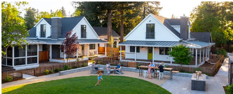
Photo: Riverhouse, Healdsburg, CA Source: https://jzmkpartners.com/project/riverhouse/
