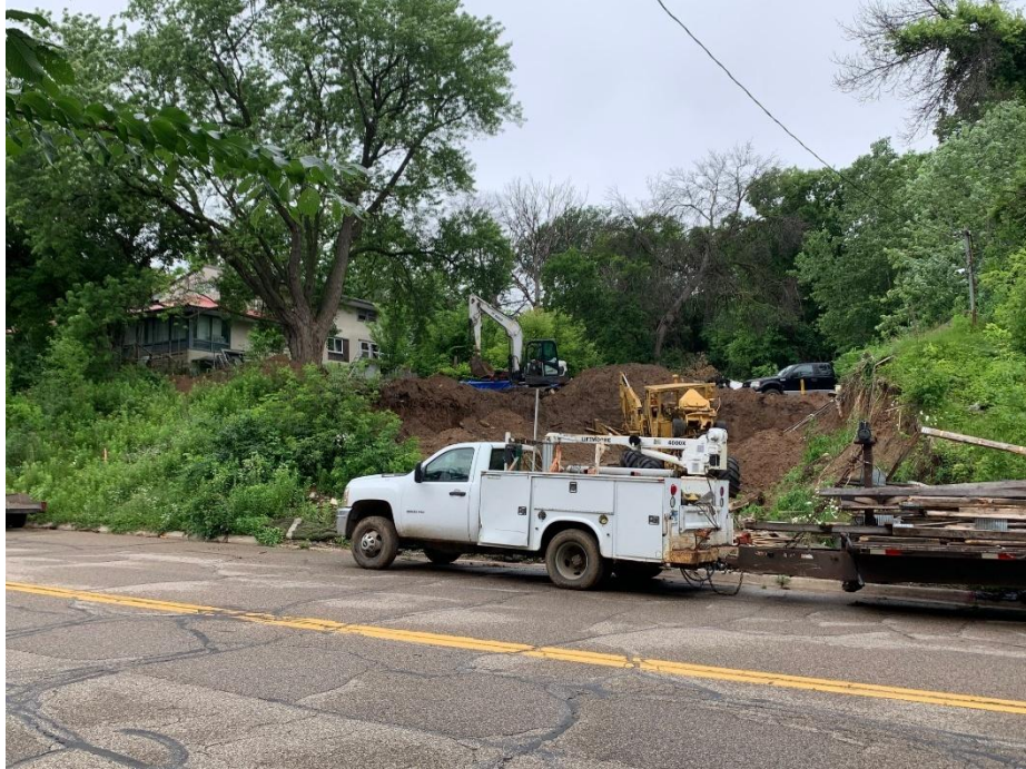
View of Demolished Home and Site of Future Twinhome at 1579 Stickney Avenue (6/26/25)
