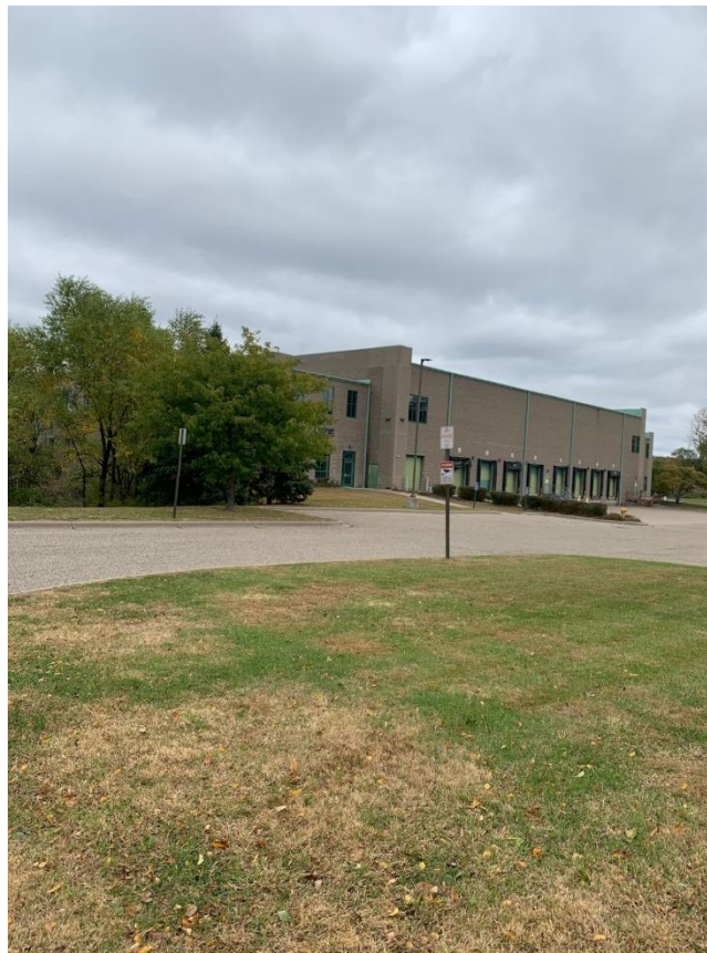
View of 205 Hardman Avenue South Building from Hardman Avenue (Photo Taken 10/22/25)
