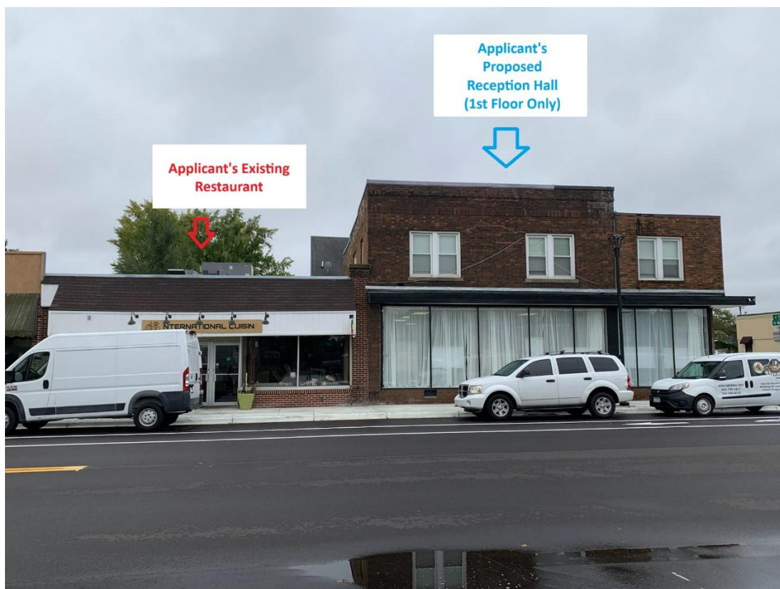
Applicant's Existing Restaurant at 417 Marie Avenue & Proposed Reception Hall at 421 Marie Avenue
