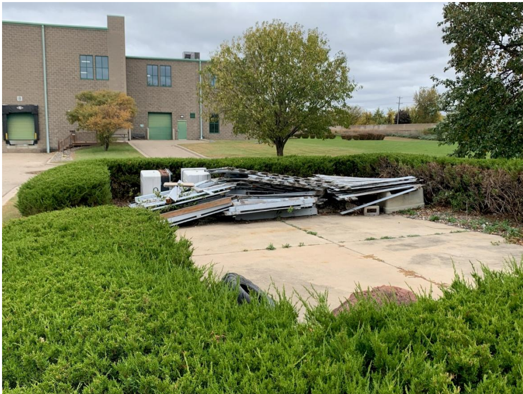
Demolished Trash Enclosure (Photo Taken 10/22/25)
