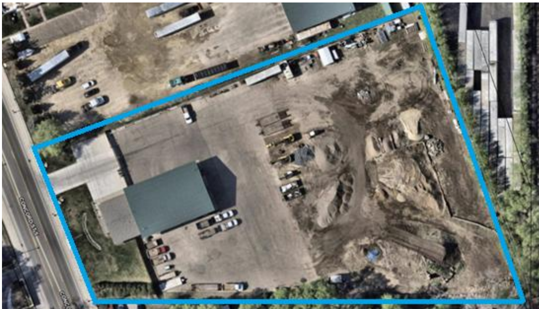
Existing Conditions at 1301 Concord Street South (Kamish Excavating)
