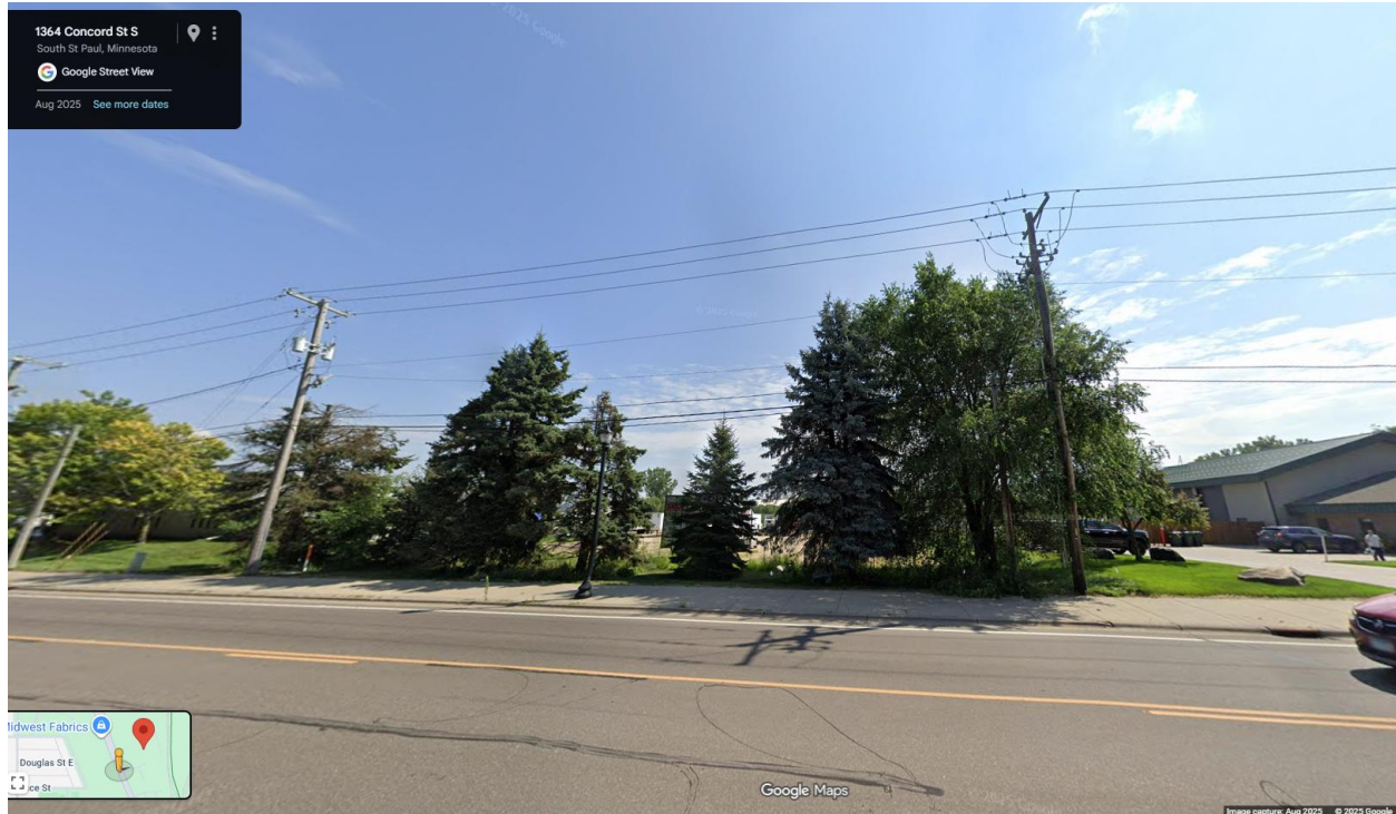
Google Streetview Photograph of the Area Between the Two Existing Buildings Where the New 6,575 Square Foot Building Would be Located
