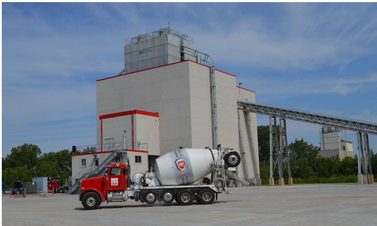
Stucco finish applied to ICF form face. Taupe color finish and red trim
