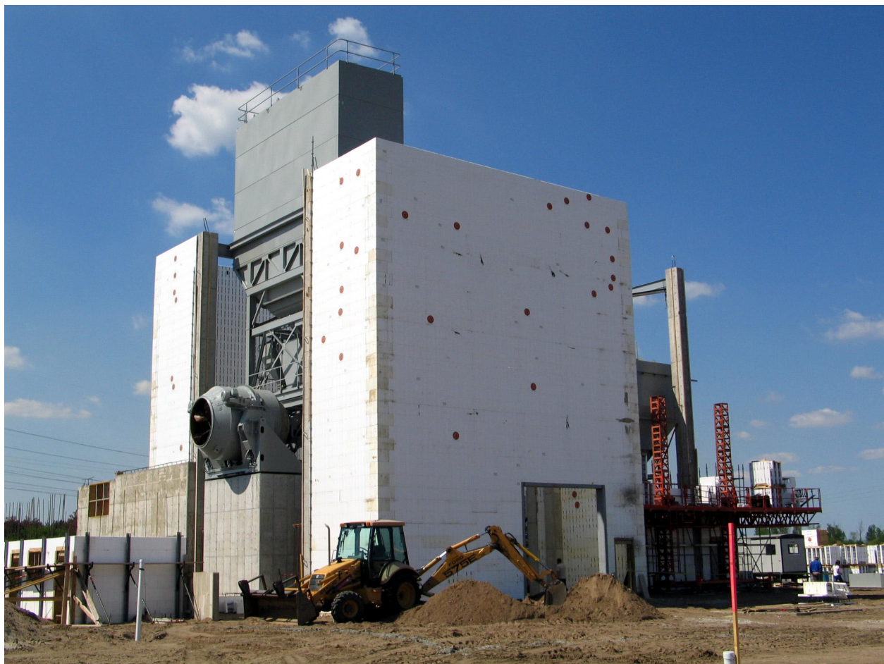
Cast-in-place structural walls and ICF forms for enclosure.
