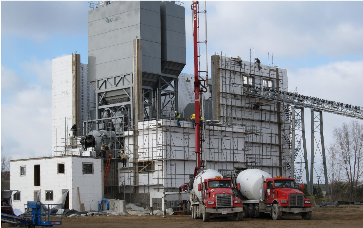
ICF plant enclosure. Walls poured in 8 foot lifts with 4000 psi concrete
