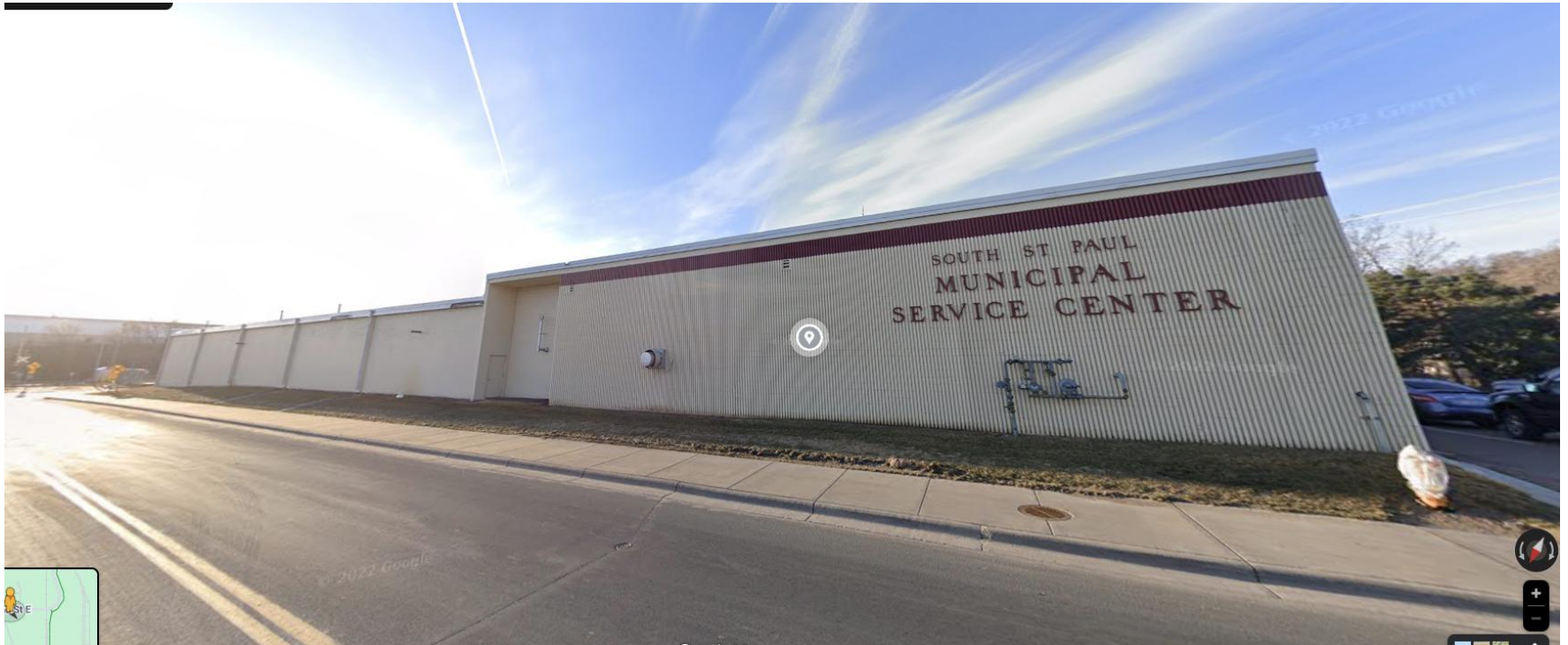
Google Streetview of Front of Existing Public Works Building (2022)
