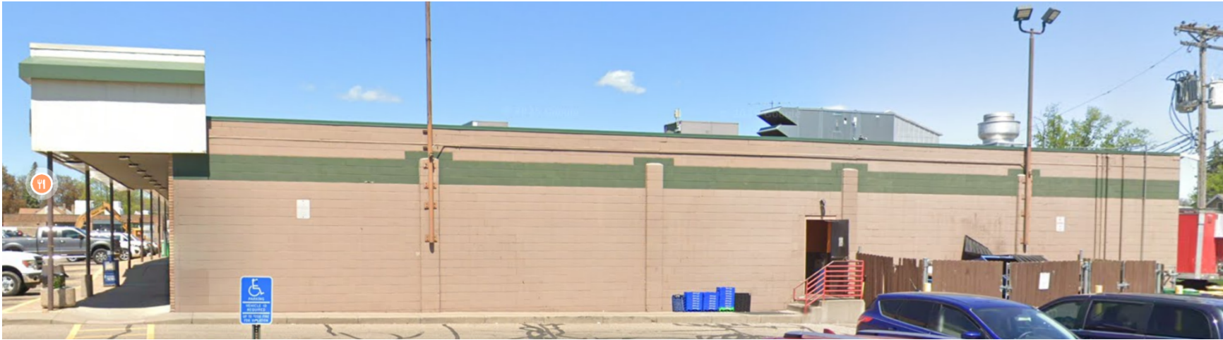
Southern Façade of Southview Shopping Center
