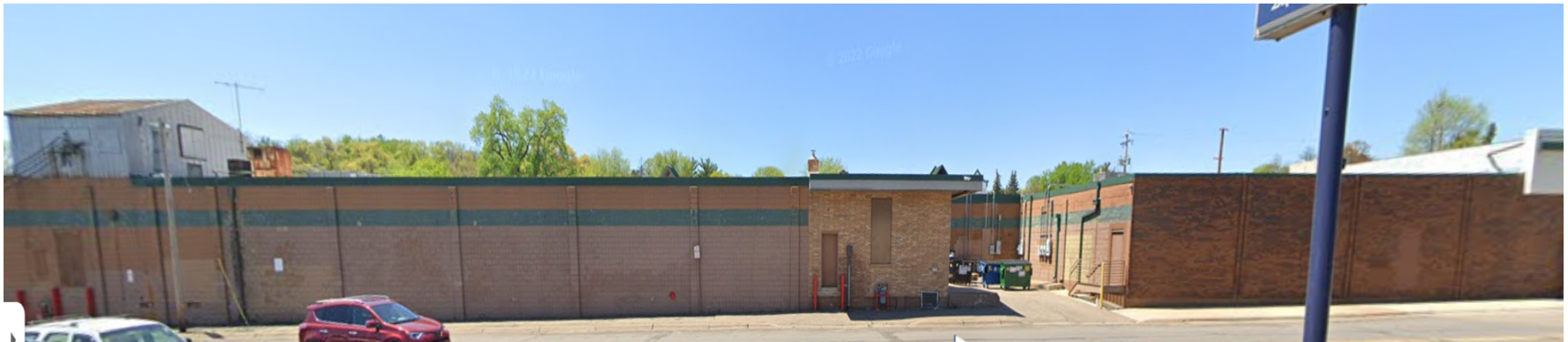
Eastern Façade of Southview Shopping Center
