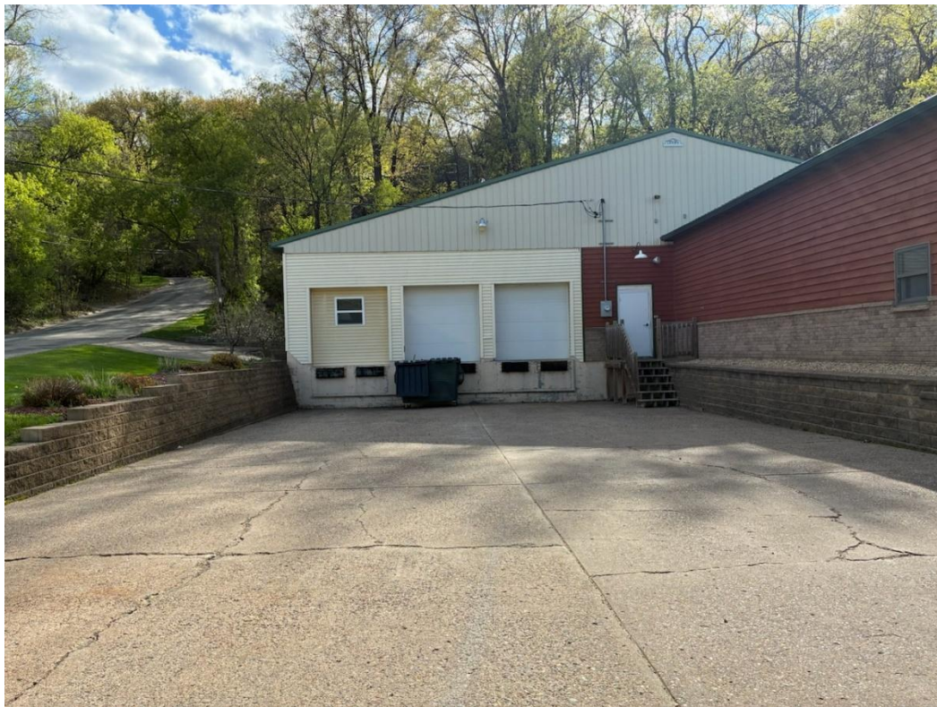
Recessed Loading Dock Area Along Concord Street
