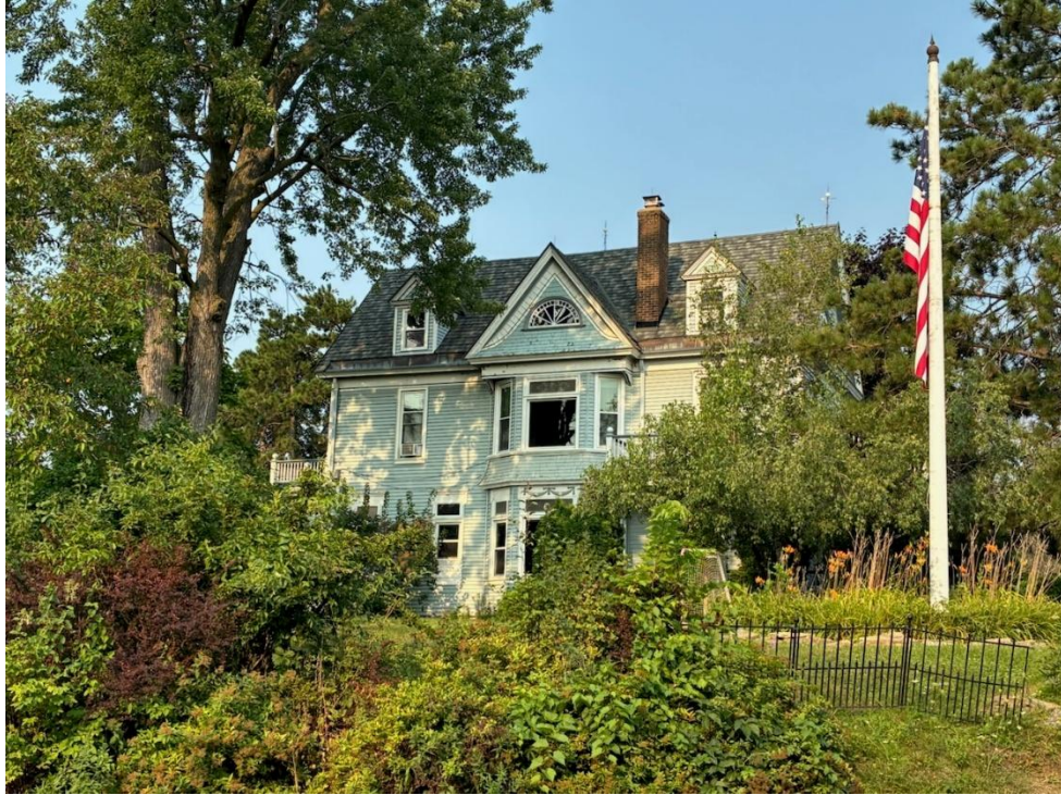
This is the side of the house that faces what is legally the front property line
